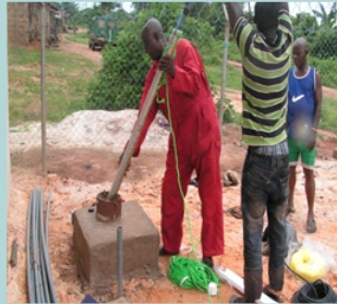
INSTALLATION AND TESTING THE SQF 2.5-2 GRUNDFOS PUMP
