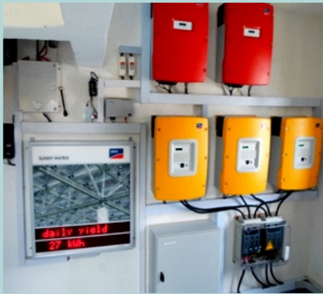
25KW SMA SOLAR HYBRID POWER STATION
