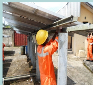
TECHNICIAN NETWORKING SOLAR ARRAYS
