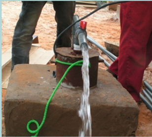
INSTALLATION AND TESTING THE SQF 2.5-2 GRUNDFOS PUMP
