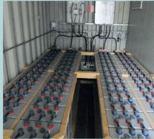
TUBULAR BATTERY BANK
