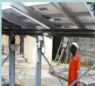
SPDC SUPERVISOR INSPECTING CONNECTIONS
