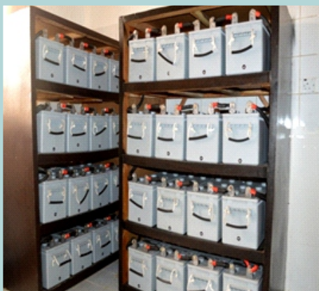
1,680Ah @48 Volts, BACK-UP BATTERY BANK
