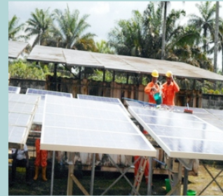
WASHING OF SOLAR PANELS
