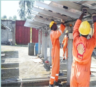
TECHNICIANS NETWORKING SOLAR ARRAYS
