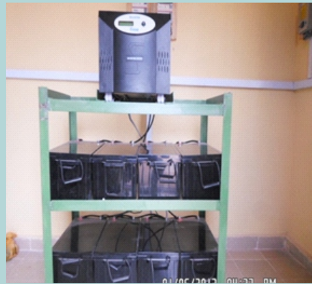
5KVA INVERTER & BATTERY BANK
