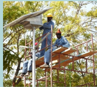
TECHNICIANS DOING INSTALLATION
