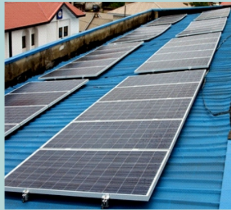
ROOF-MOUNT SOLAR ARRAY
