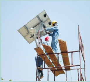
TECHNICIANS DOING INSTALLATION
