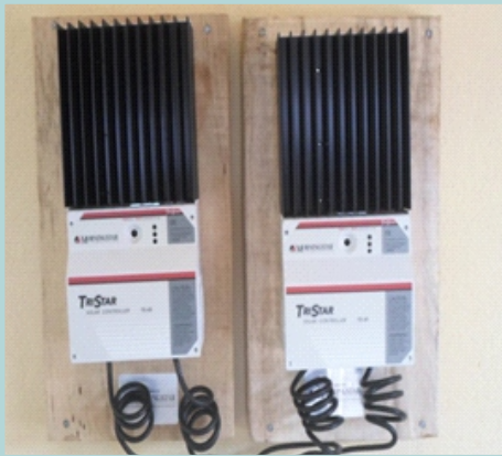
SOLAR CHARGE CONTROLLER
